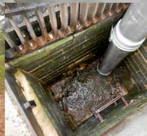
Powaboom option cleaning catch basin.
